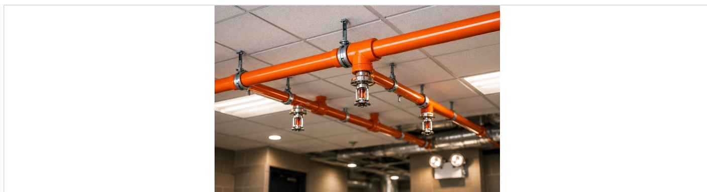
Orange CPVC fire sprinkler pipework — lightweight and fast to install, but vulnerable to chemical contamination from adjacent materials.
